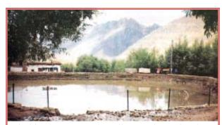
A kul leads to a circular village tank, as the above in the Kaza village, from which water is released as and when required.
